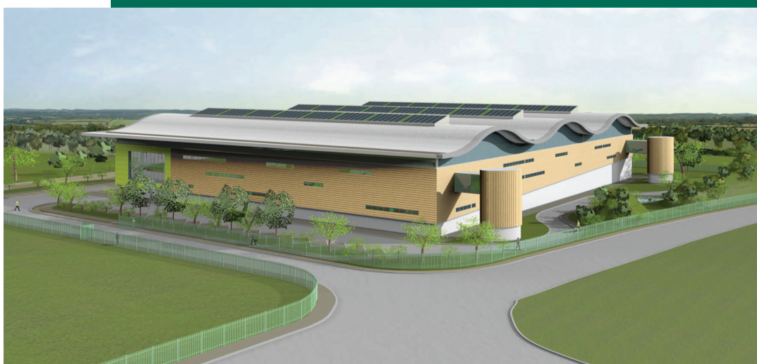
Construction work at Gillmoss should be completed by 2010
